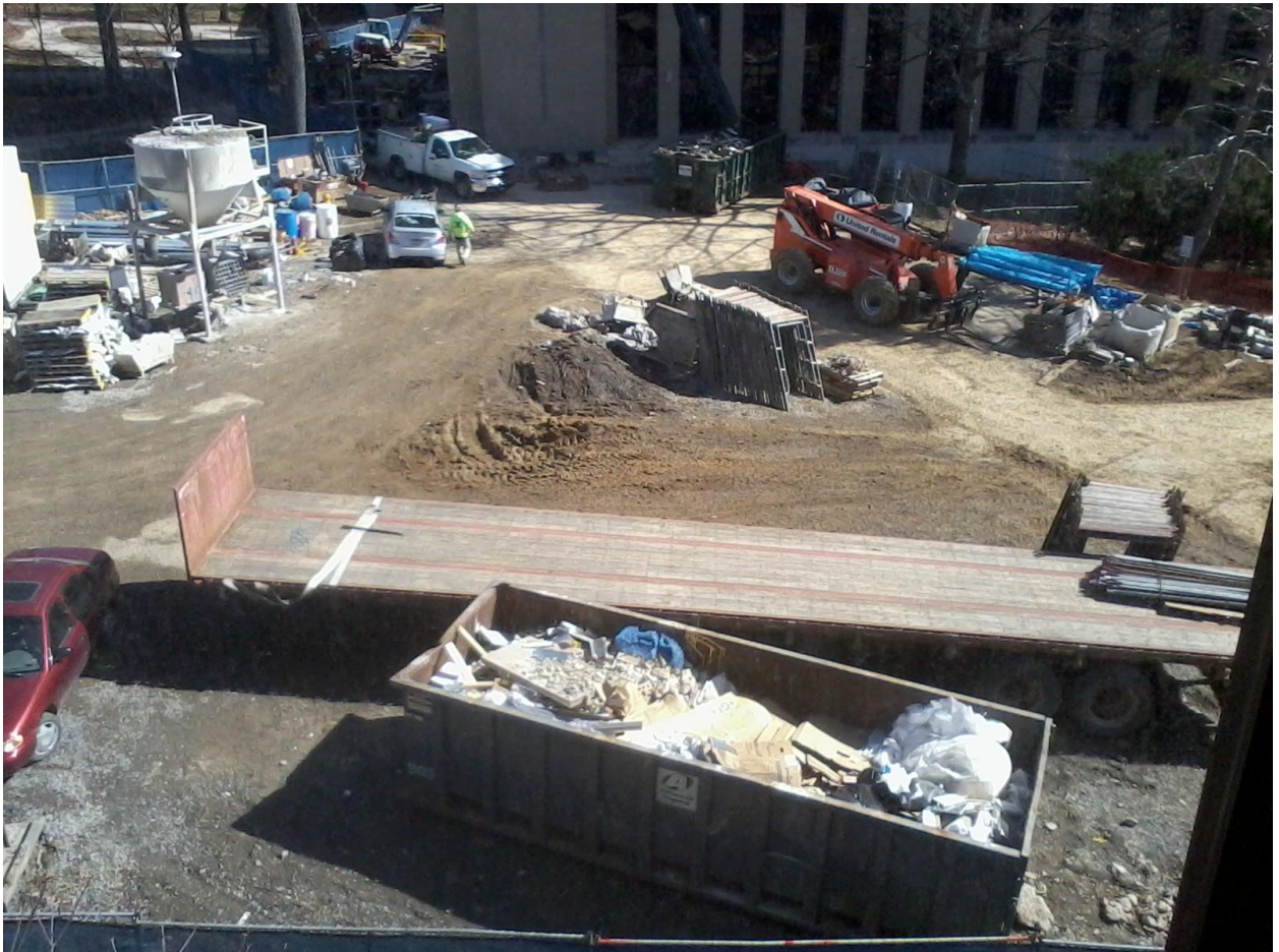
Figure 21: Dumpsters on the worksite.
