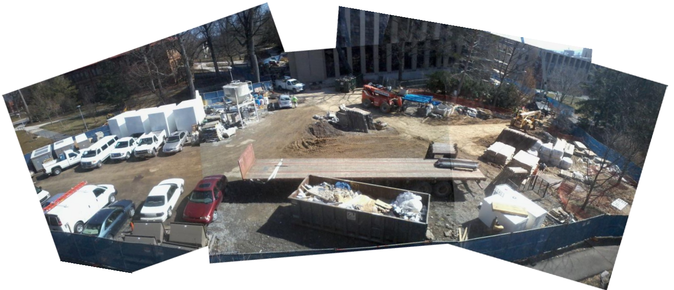
Figure 13: Panorama of existing job site.
