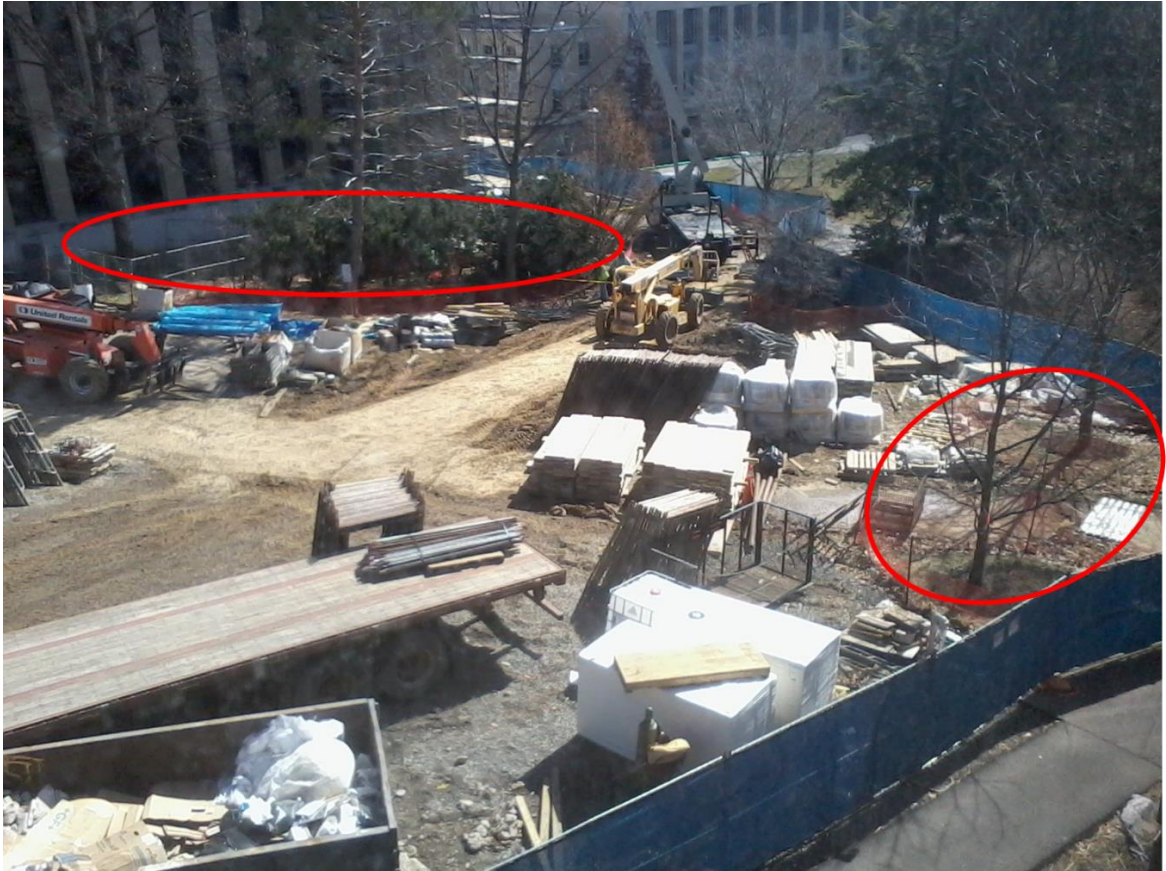
Figure 9: Fenced in areas with trees to be protected.
