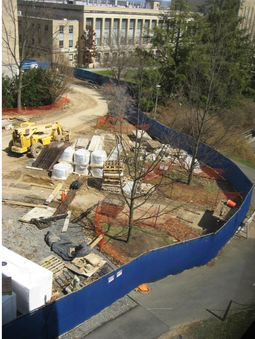
Figure 10: Material storage on slope.
